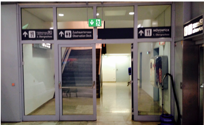
Fig. 2: Typical marking of escape routes and emergency exits
