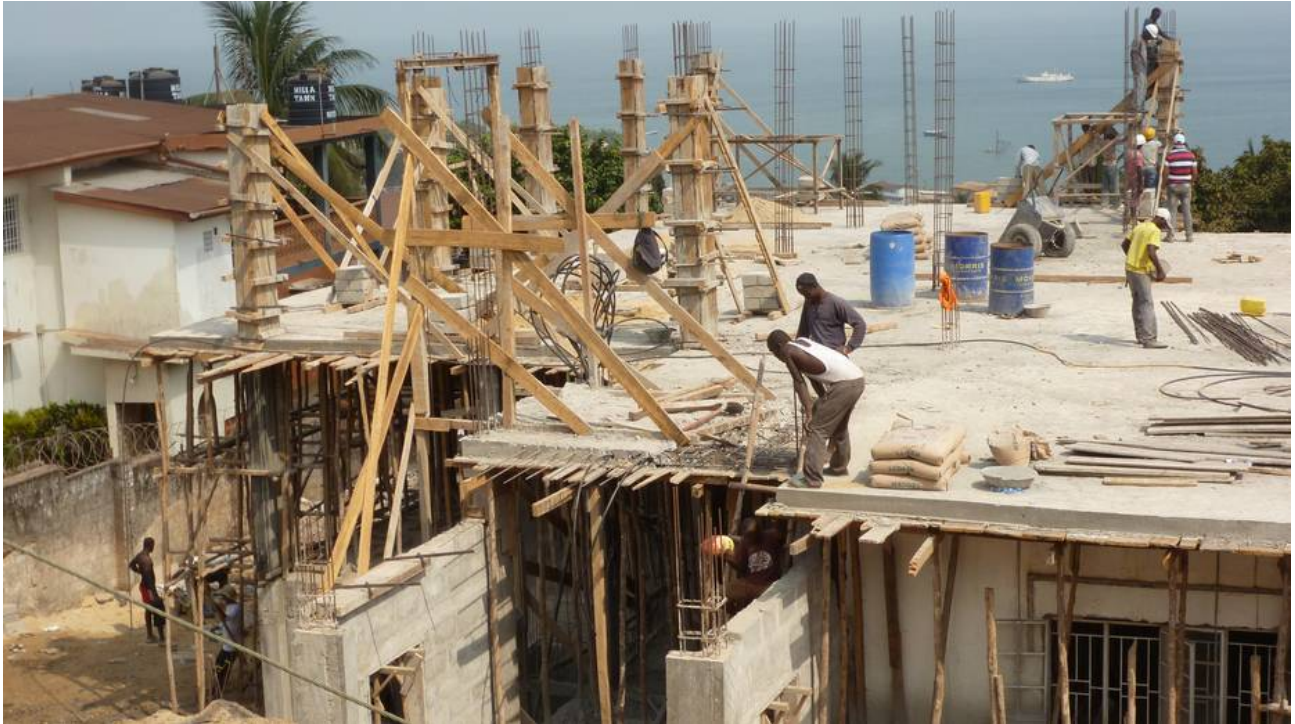
Baustelle in Freetown © Juliane Westphal
